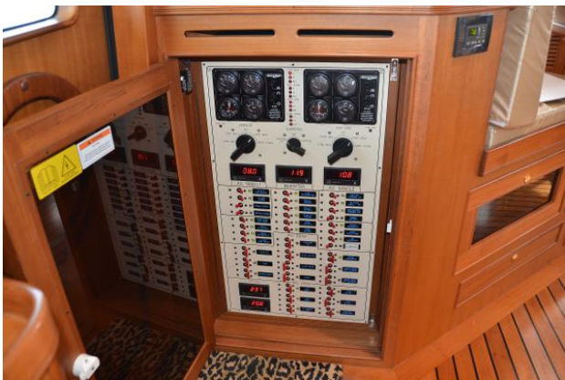
Main Electrical Panel
