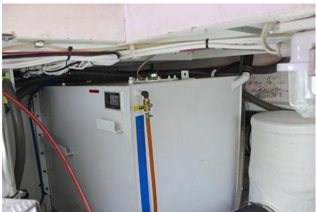
Port fuel tank
